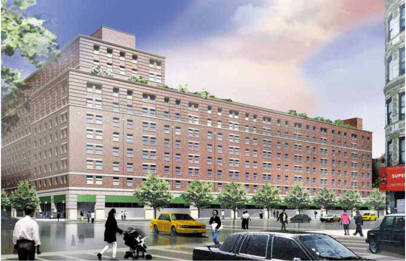
The Central Harlem Renaissance Plaza project in New York City used precast concrete hollowcore slabs for its flooring units due to the material's speed of construction, economy, fire resistance, long span capability and acoustical control. Illustration: Greenberg Farrow Architecture Engineering Development
